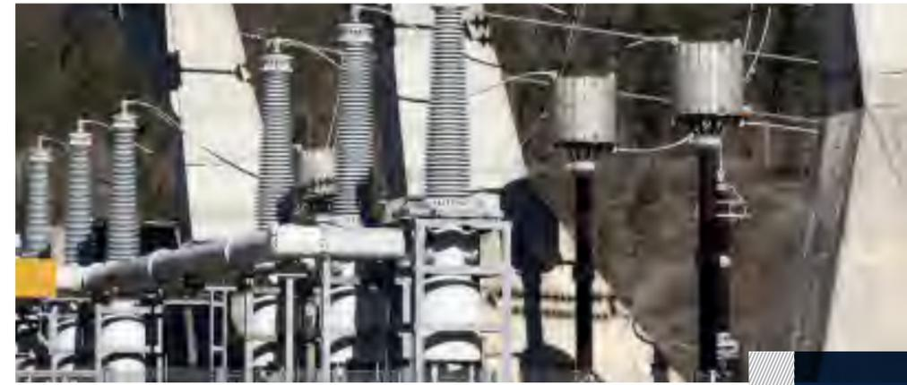
Neutral grounding resistors have a number of advantages that have ended up replacing insulated neutral and reactance grounding distribution systems. The most interesting advantages attributed to grounding resistors are:
